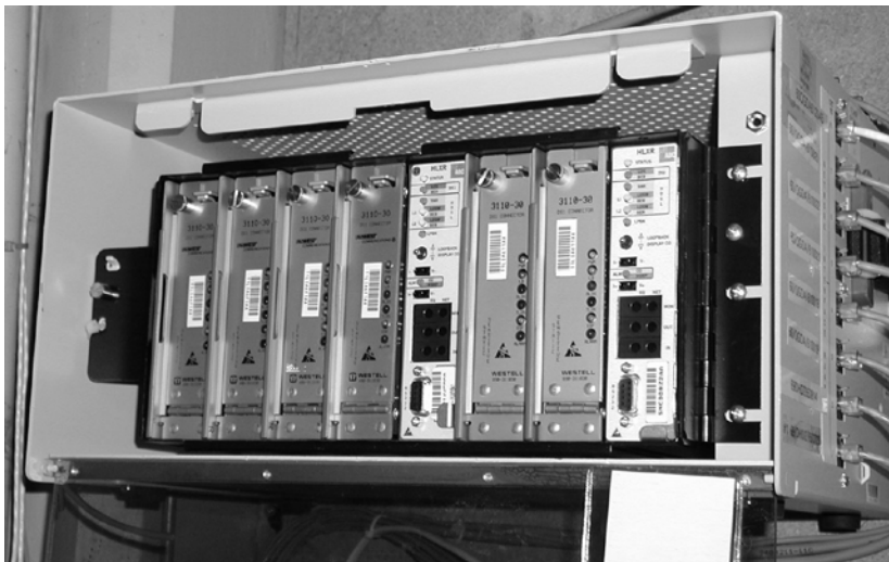
Figure C.39 CSU (Channel Service Unit)
