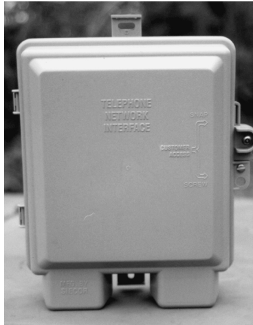
Figure S.12 SNI (Standard Network Interface)
