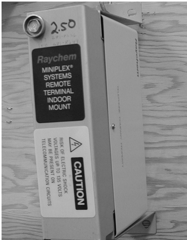
Figure U.2 UDC (Universal Digital Carrier) Remote Unit
