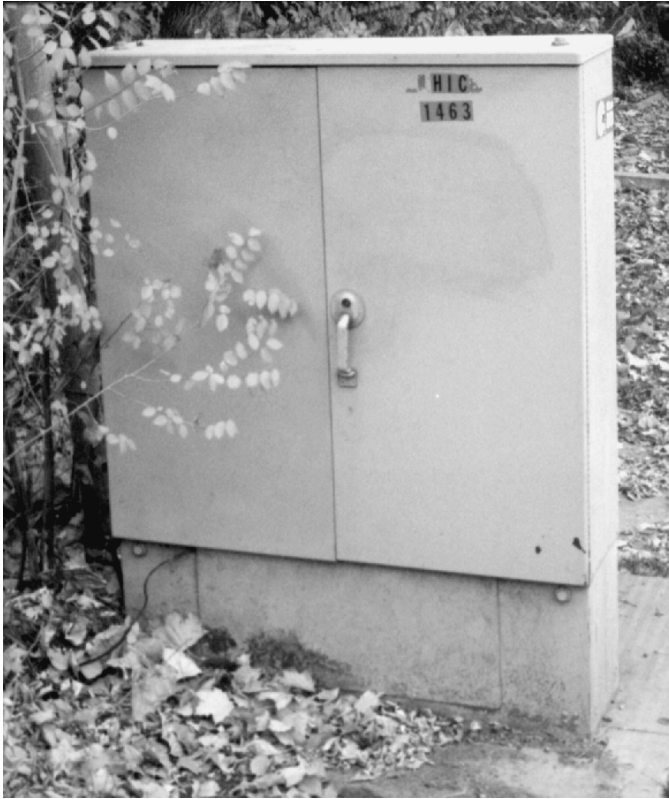
Figure A.3 Access Point (AP) Cross Box
