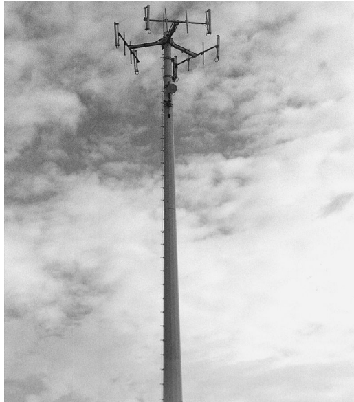
Figure M.15 Monopole Antenna With PCS/Cellular Antenna Array
